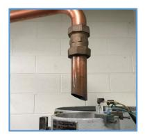
Air Gap = An air gap is a physical unobstructed separation through free atmosphere between the free-flowing discharge end of any pipe or outlet supplying potable water and the flood-level rim of a receiving receptacle. The air gap, when maintained and inspected, is the most reliable means of protection because it is not subject to any mechanical failure. A common air gap in a plumbing system are bathtubs, swimming pool fills, and sinks.
